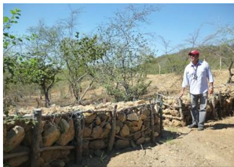
Figure 11: National Environmental authorities from MINEC provided technical and financial support to rural communities to develop artisanal ditches in Tupure river basin, one of the tributaries of Maticora river, in north-western Venezuelan Falcón state, in order to stop erosion and promote soil and vegetation recovery.
